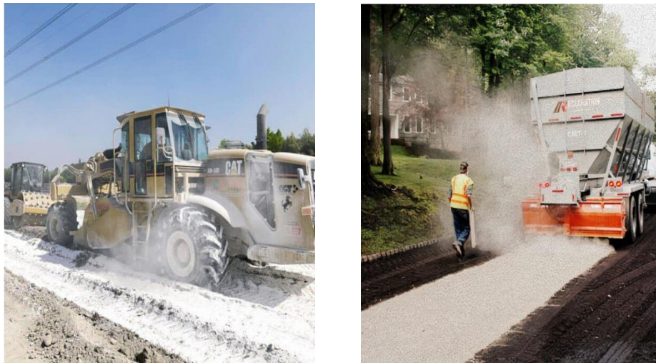
Figure 2 (a) Subgrade stabilization by cement (b) Subgrade stabilization by Lime
